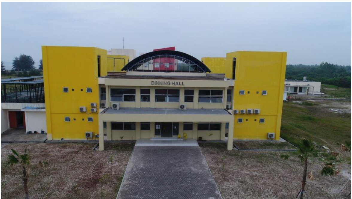
Gambar 2.18 Gedung Dinning Hall
