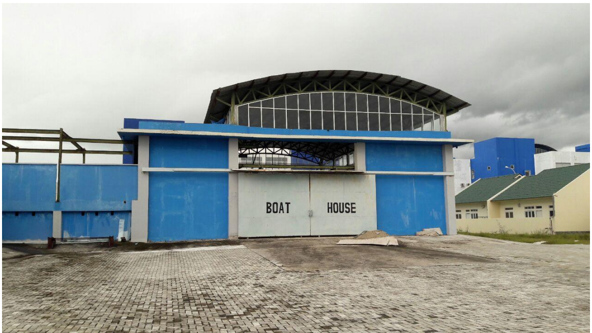
Gambar 2.16 Gedung Boat House
